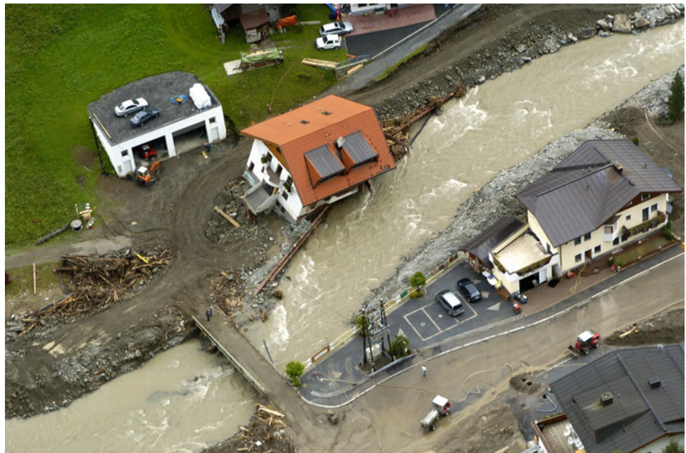
Fig. 6.3 Dynamic flooding of Trisanna river in Kappl, Austria, after the flood events of August 2005. Picture credits Austrian Armed Forces, with permission
