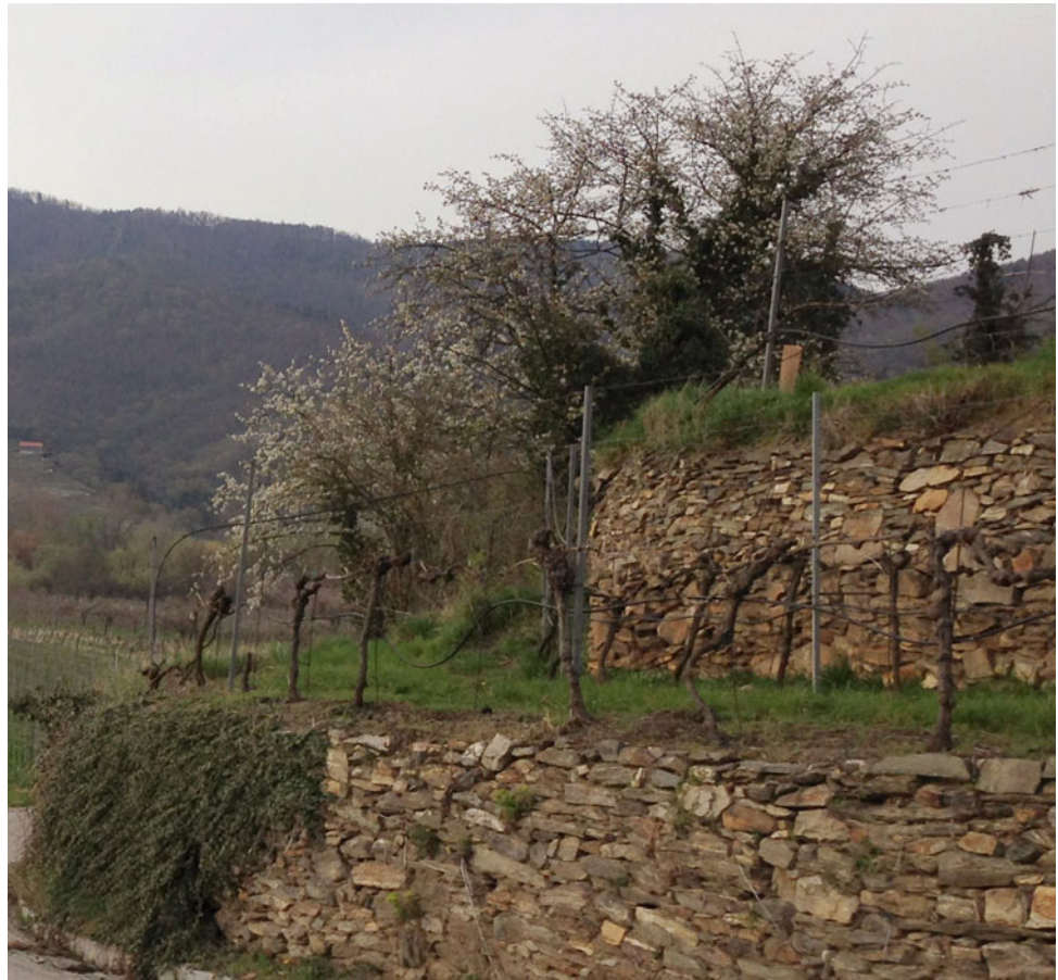
Fig. 10.9 Dry masonry walls in the Wachau near Arnsdorf. Photo: D. Riedl
