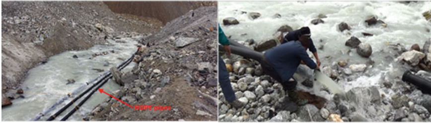
Fig. 8.4 GLOF mitigation (siphoning of impounded water) at South Lhonak Lake in 2016
