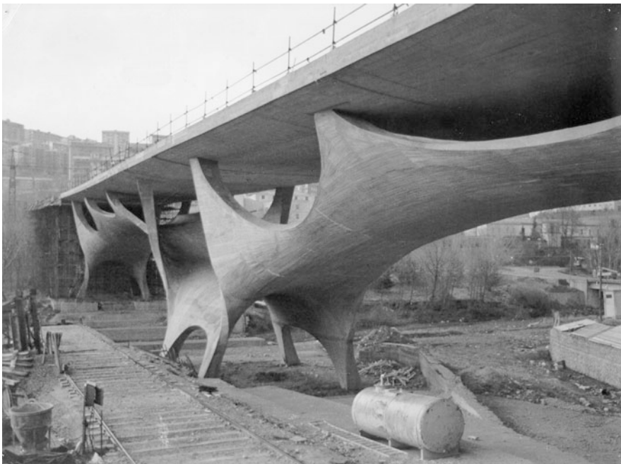
Fig. 21 Bridge over the Basento river in Potenza, 1967–1975, S. Musmeci: The indelible traces left by the wooden formwork on the shell. Courtesy MAXXI Architecture Archive (SIXXIdata)
