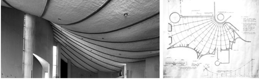
Fig. 13 The Sant'Alberto Church at Sarteano, Siena, 1969–1972, S. Musmeci, G. Petrangeli: (left) Inside view; (right) The plan. Courtesy MAXXI Architecture Archive (SIXXIdata)
