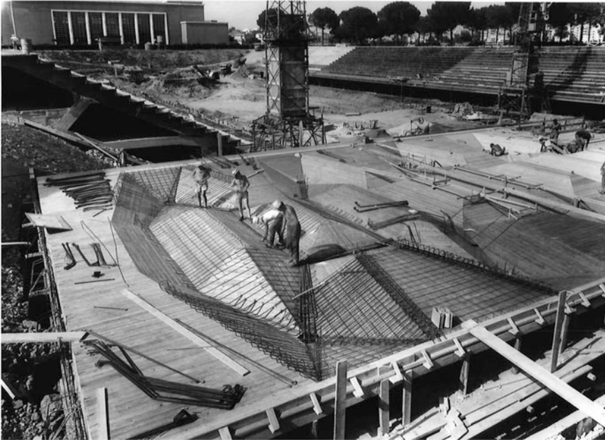
Fig. 3 The roofing of the Restaurant for the Swimming Stadium, 1958, S. Musmeci, A. Vitellozzi. Courtesy Coni Archive (SIXXIdata)
