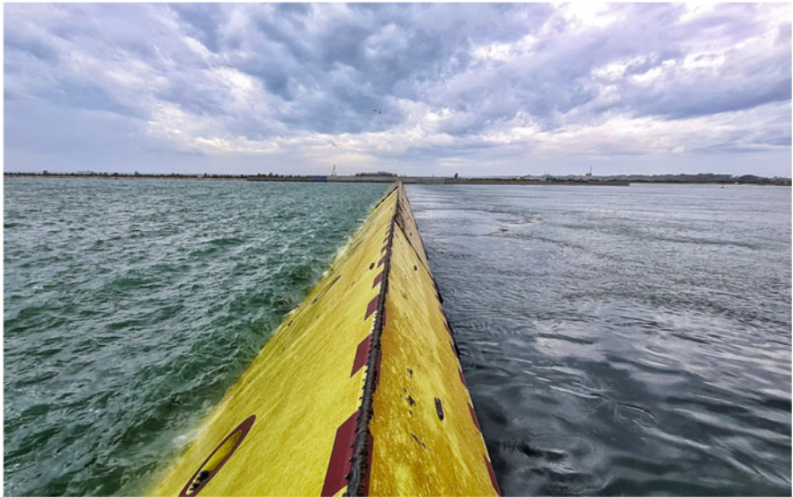
Fig. 10 MOSE Project, Venezia, © by permission. October 3, 2020. At 9:52 all MOSE 78 gates isolated the lagoon from the sea. In the town, the tide level settled at around 70 centimeters, while the gates blocked the sea at 125 centimeters. To the left the open sea, to the right the lagoon
