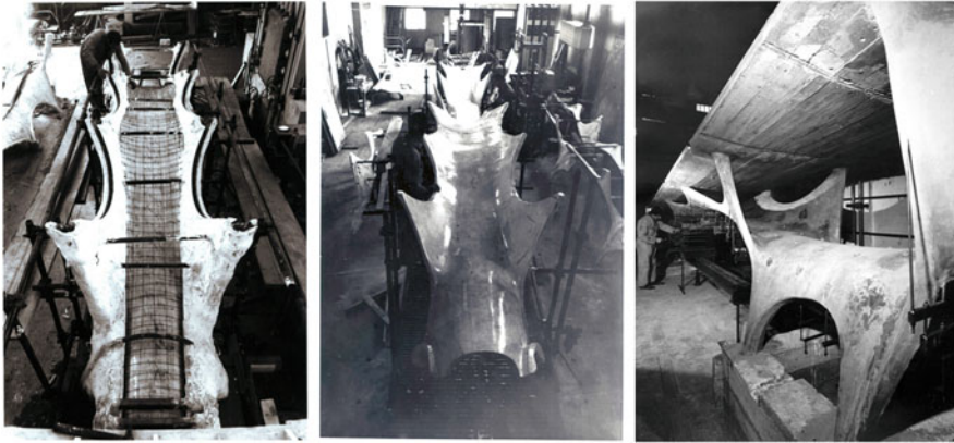
Fig. 19 Bridge over the Basento river in Potenza, 1967–1975, S. Musmeci: Microbeton model, 1:10, 1970–1971. Courtesy ISMES Archive (SIXXIdata)
