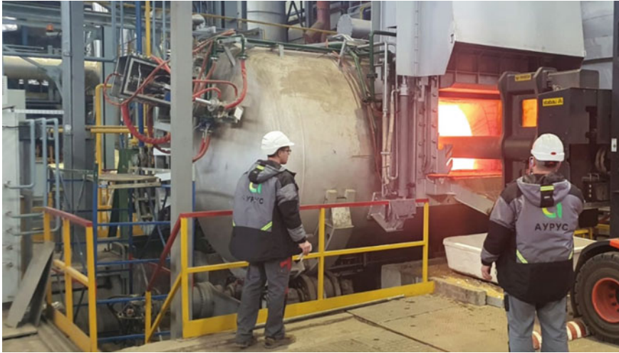
Fig. 5 Anode furnace at Aurus during operation
