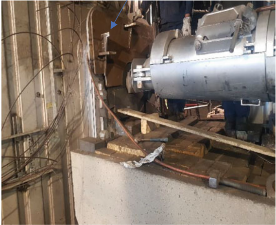
Tap-hole arch holding plate installed
