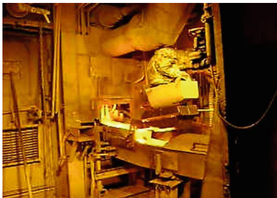
Fig. 8 Robot operating jackhammer tap-hole opening tool
