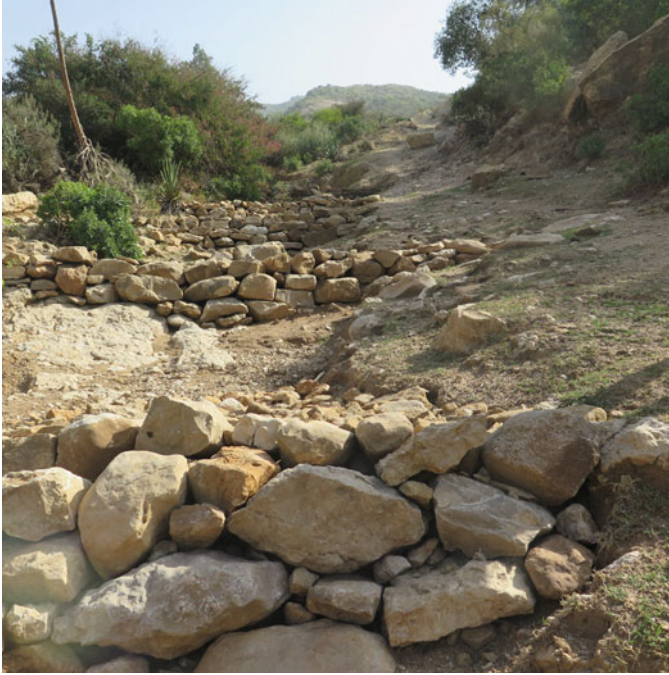
Fig. 26.3 Newly constructed check dams in an outwash area in Abreha we Atsbeha. (Photo: E. Sigman)
