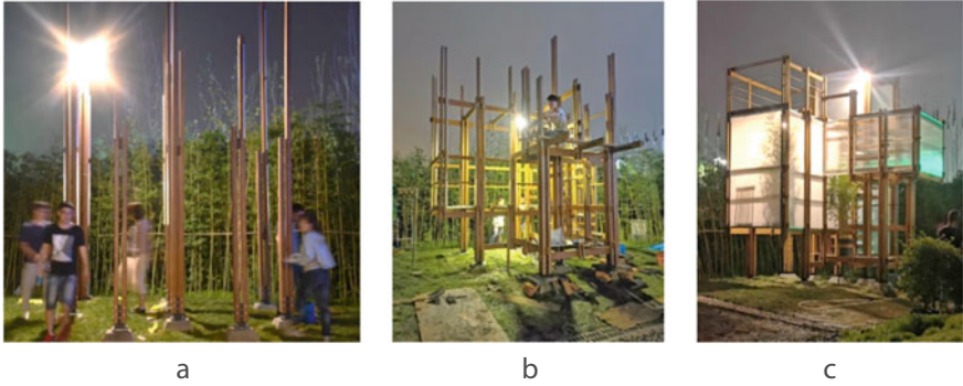
Fig. 12 Different stages of assembling on-site. Day 1 (a); Day 2 (b); Day 3 (c)
