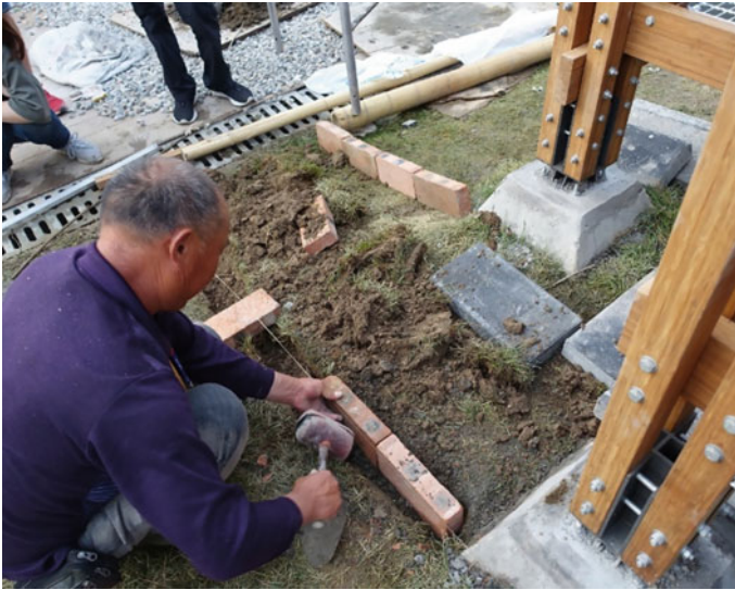
Fig. 15 Red brick drawing the edge at the entrance tread
