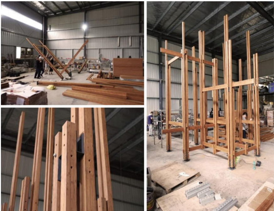
Fig. 11 Pre-construction in the factory
