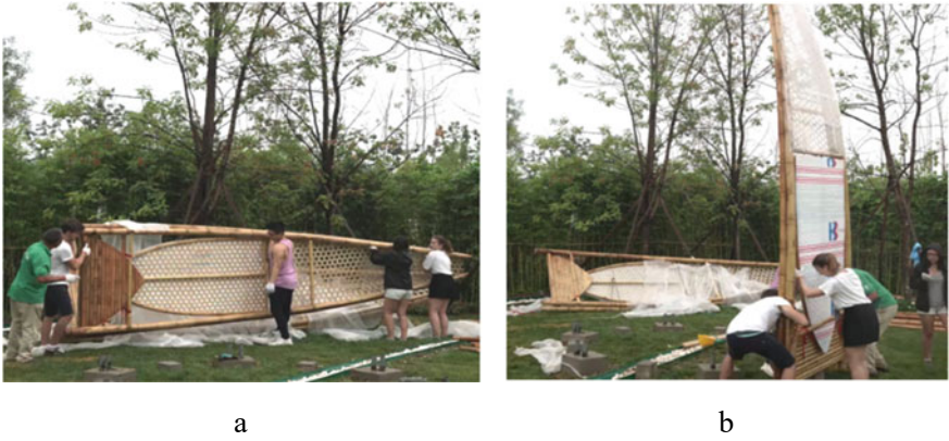
Fig. 10 Module preparation (a); initial module installation (b)
