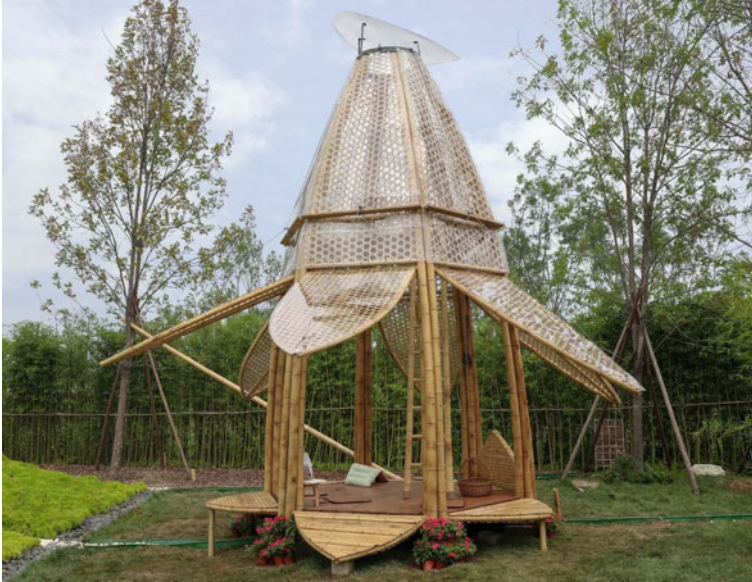
Fig. 15 Final look of the constructed pavilion
