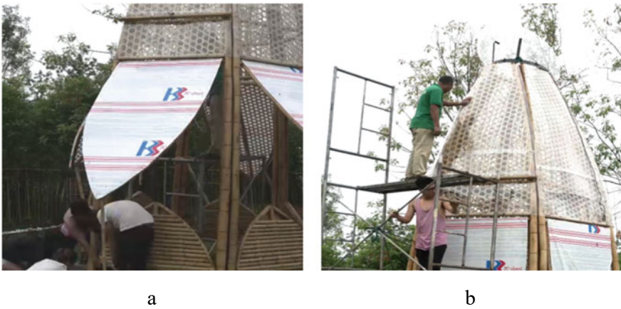
Fig. 12 Adjacent module connection (a); installation of ceiling element (b)
