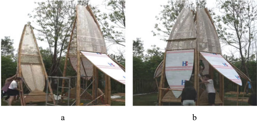
Fig. 11 Adjacent module installation (a); complete the modules (b)
