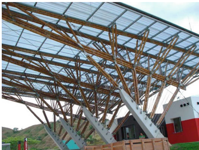
Fig. 4 Cable-stayed bamboo cantilever, toll gate in Armenia, Colombia. Photo by: Forgemind ArchiMedia [48]
