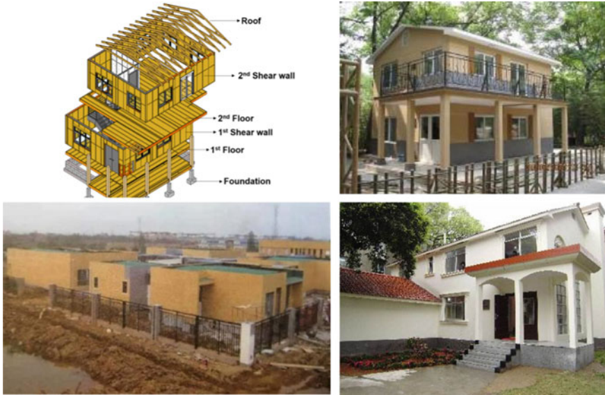
Fig. 8 Lightweight GluBam frame constructions
