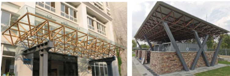
Fig. 14 Hybrid bamboo-steel truss
