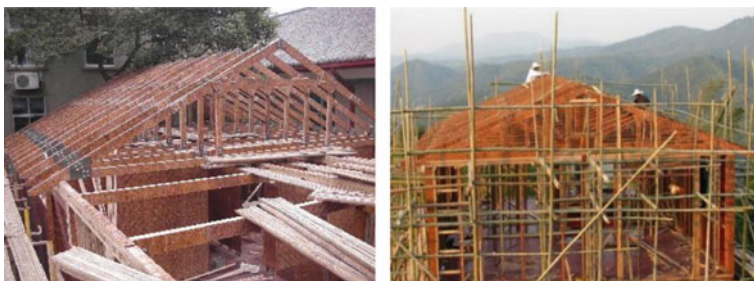
Fig. 11 Roof system in lightweight GluBam structure
