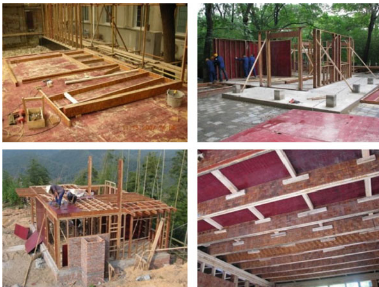
Fig. 10 Processing and installation of lightweight GluBam shear wall and floor diaphragm
