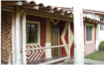
a. Bahareque bamboo house in Colombia
