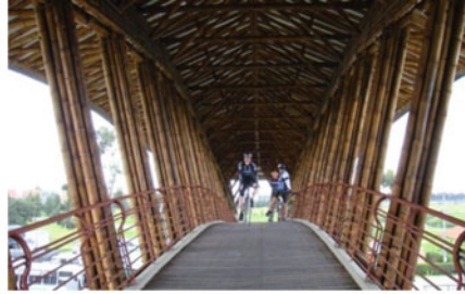
b. Jenny Garzon Bridge in Colombia. (photo by Liu Kewei)
