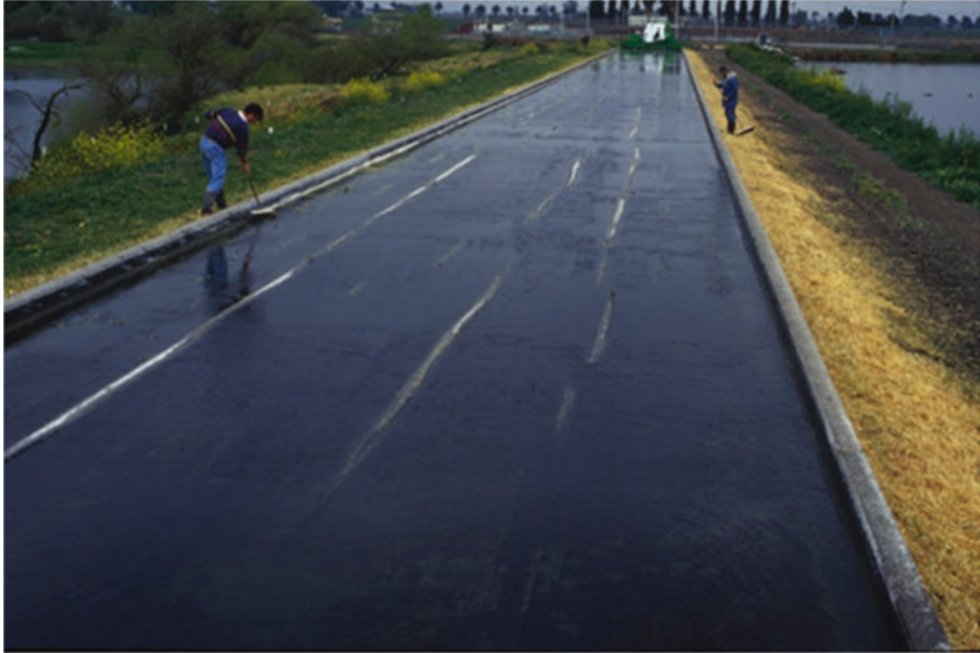
Fig. 23.3 First large-scale algal turf scrubber (ATS) system at the Patterson municipal wastewater treatment plant, California. (Photo courtesy Rupert J. Craggs). ATS improves water quality by passing a shallow stream of wastewater over the surface of a gently sloped flow-way (Craggs 2001). The system was 154.2 m long and 6.5 m wide, producing up to 62 g/m per day. Mat forming species were mainly cyanobacteria (mostly Oscillatoria ), with canopy of filamentous algae ( Ulothrix sp. and Stigeoclonium sp. prevailing in the summer) and diatoms (Craggs 2001)
