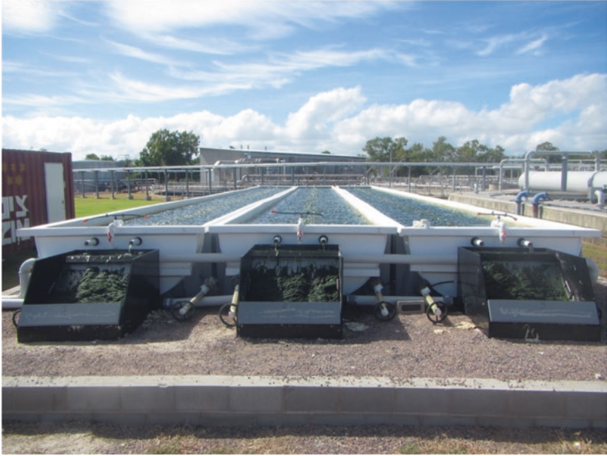
Fig. 23.2 Wastewater treatment pond for macroalgae cultivation in Townsville, Australia. (Photo courtesy of Andrew J. Cole): Oedogonium sp. was cultivated in the treated municipal wastewater containing mean concentrations of approximately 4 \text{ mg} \cdot \text{l}^{-1} N and 0.8 \text{ mg} \cdot \text{l}^{-1} P (Cole et al. 2016a). Over a 12-months period, a tertiary treatment by Oedogonium reduced the concentrations of total N and P by 36% and 68%, resulting in 491 kg DW which recovered 24.4 kg N and 4.8 kg P. The algae were used as the feedstock to produce compost and biochar (Cole et al. 2016b)
