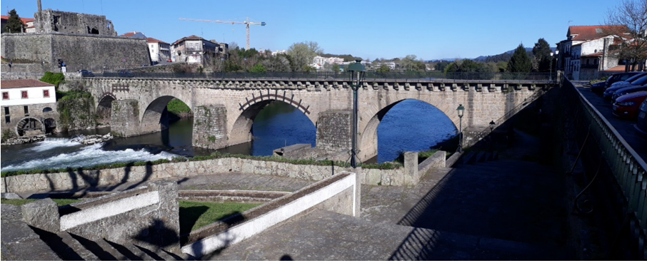
Fig. 1. Barcelos Bridge (downstream view).
