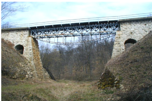
Fig. 3. The Rátót viaduct with stone masonry abutments
