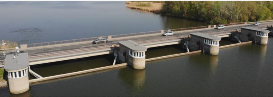
Fig. 1. Side view of the analyzed bridge.
