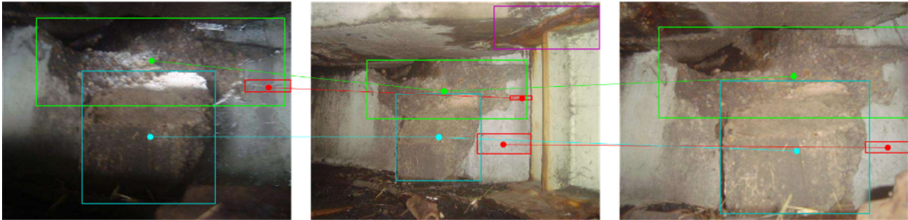
Fig. 4. Defect matching example. Different defect types are drawn in different colors. Defect matching is performed between all relevant image pairs. Multiple instances of the same defect were correctly matched across different non-UAV images. Red bounding boxes represent detected cracks. Red lines between images indicate that the defects were matched.
