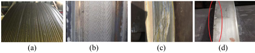
Fig. 25.2 Types of wear in the rotary kiln tyres [9]: a groove-type pattern when the drum is out of alignment; b spalling-type pattern due to excessive wheel skewing; c gouging-type wear from obstruction on the tyre; d wear due to lubrication penetration into metal causing cracks
