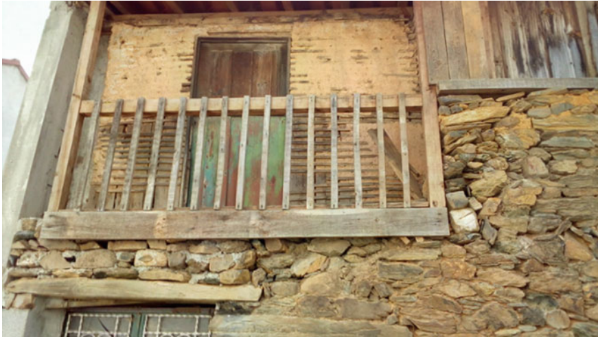
Fig. 9.2 Example of a two floors Tabique dwelling of this region
