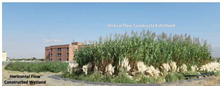
Fig. 23.1 The demonstration constructed wetland system at the Neyshabor University in Iran for dormitory wastewater treatment
