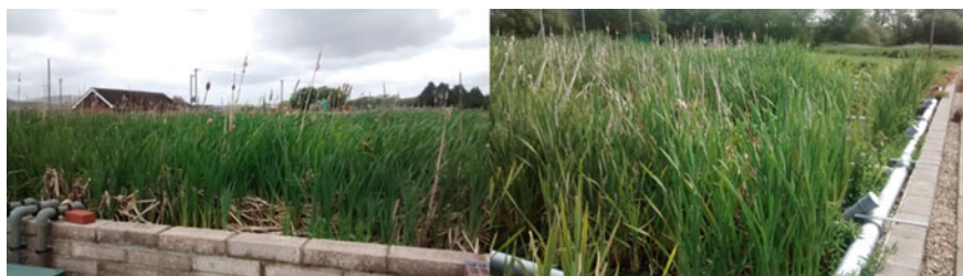
Fig. 23.3 Pictures of the research aerated VFCW system at Petersfield WWTP in the UK
