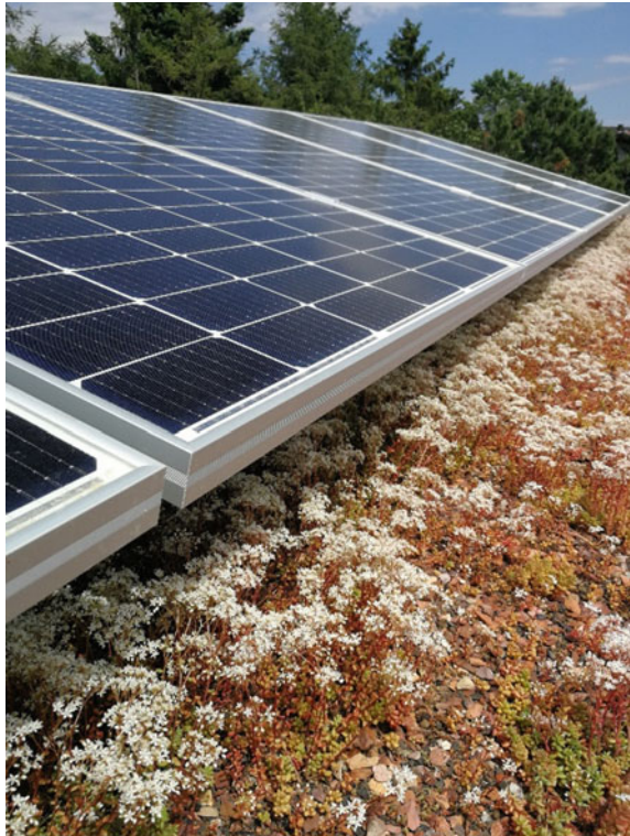
Fig. 18.3 The combination of green roof and energy production yield synergies ©GRÜNSTATGRAU
