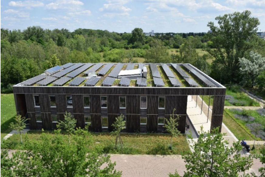
Fig. 18.4 Solargreen Roofs increases biodiversity through different shading areas © Bundesverband GebäudeGrün e. V. (BuGG)
