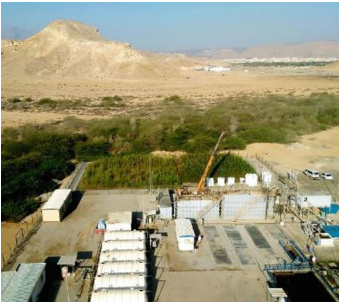
Fig. 23.2 Aerial picture of the full-scale research VFCW facility at the conventional wastewater treatment plant in Quriyat, Oman
