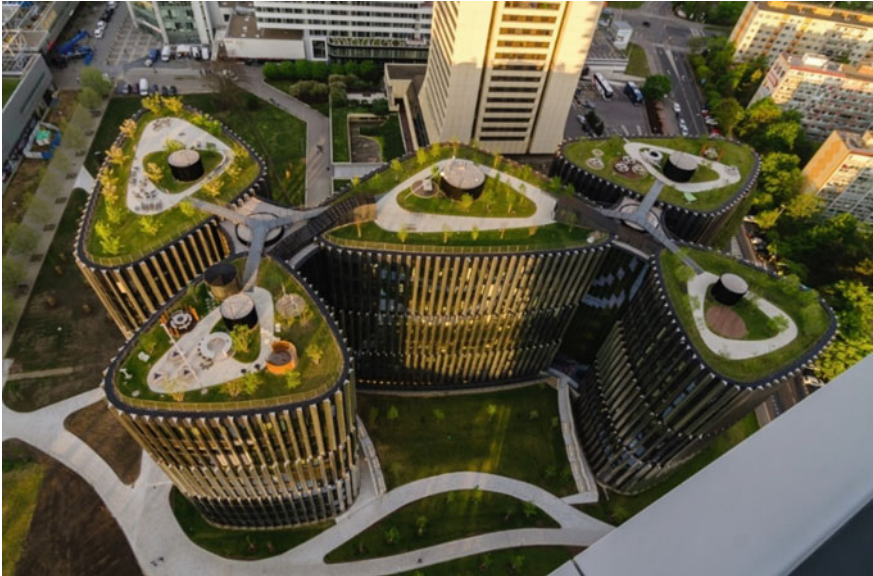
Fig. 18.2 An intensive green roof can be designed with trees ©DAM.architekti
