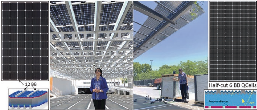
Fig. 7 Bifacial horizontal roof top solar arrays using 12 multi-busbar mono-Si modules (left); inclined half-cut 6 busbar Q-cells panels (right) under installation at Bishop Ranch, California. Single panel and cell schematics are shown. (Photo courtesy Distributed Solar Development)
