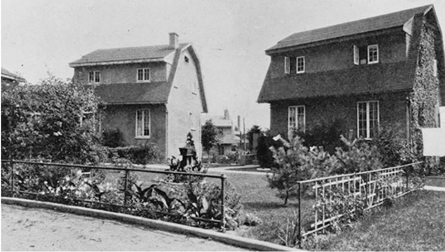
Fig. 3 Homes in Concrest (1930s). (Courtesy of the Village of East Rochester)
