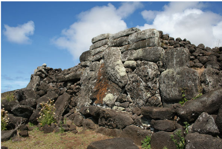
Fig. 10.6 Ahu Maitaki te Moa. A completed statue is incorporated into the back wall of the ahu
