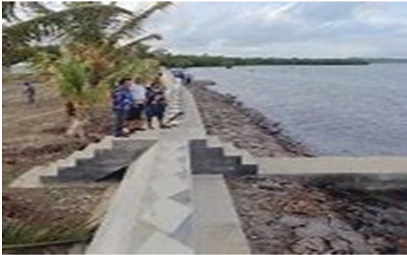
Fig. 4.5 Construction of the sea wall
