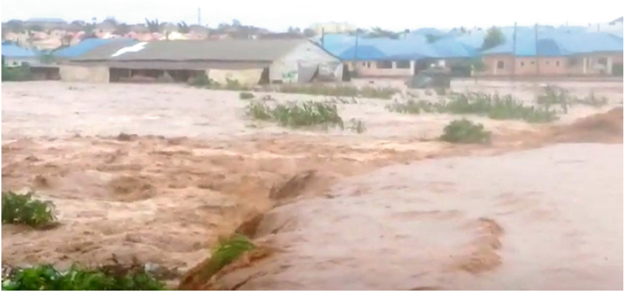
Fig. 1. Lokogoma Estate Abuja after a flood in September 2019. Source: Authors Field work, 2019.
