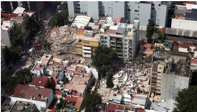
Fig. 3.5 Damage in Mexico City, Mexico
