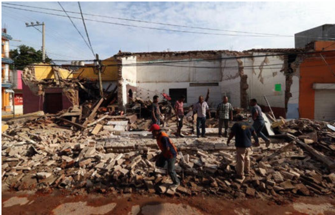
Fig. 3.4 Damages in Juchitan, Oaxaca
