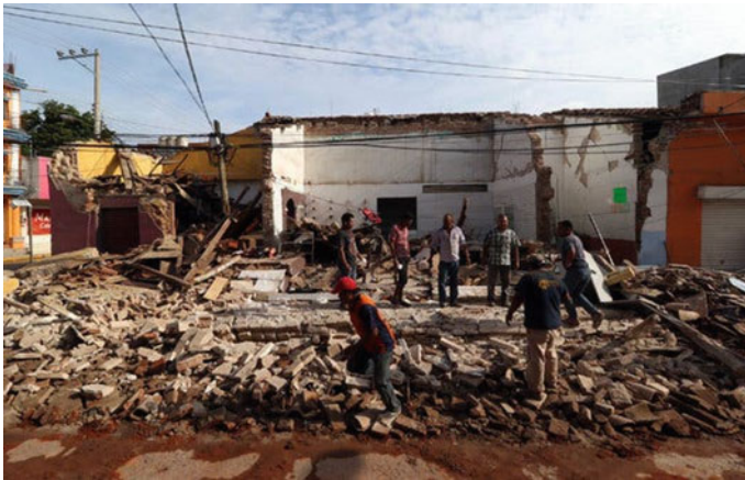
Fig. 3.4 Damages in Juchitan, Oaxaca
