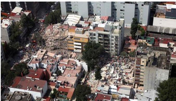
Fig. 3.5 Damage in Mexico City, Mexico
