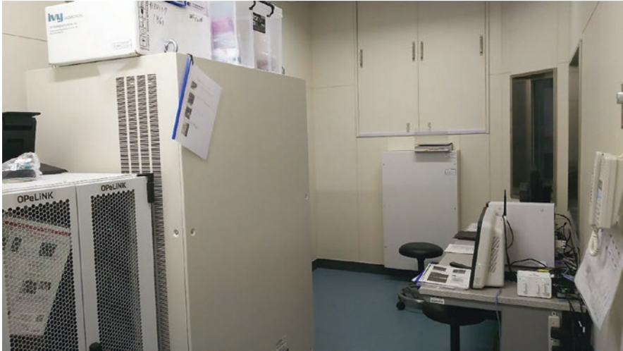
Fig. 4 Control room beside the SCOT operation room; MRI control desk on the right side, OPeLinK server on the left. The cable connecting the OPeLinK server and each item of apparatus is built within the central wall to avoid interference with the intraoperative MRI. The connecting system is not Wi-Fi; an Ethernet cable is used
