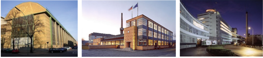
Fig. 4. AEG Turbine Factory in Berlin by Peter Behrens studio (left) Doris Antony, Berlin, Germany; Fagus pencil case Factory in Alfeld on the Leine by W. Gropius/A. Meyer in (middle) Carsten Janssen (Jaeggi 1998); and Van Nellefabriek in Rotterdam by Johannes-Andreas Brinkman and Leendert-Cornelis van der Vlugt.
