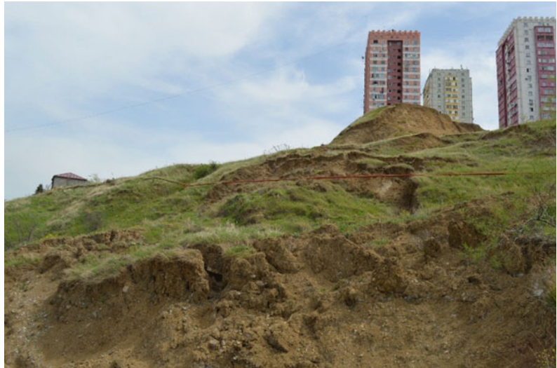
Fig. 7.6 Landslide in Sheshelidze str. (Tbilisi), April 2016 (Photo by G. Gaprindashvili)
