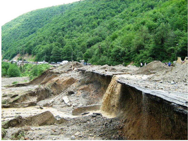
Fig. 7.5 Debris flow in Rikoti Pass (Khashuri Municipality), June 2011 (Photo by G. Gaprindashvili)
