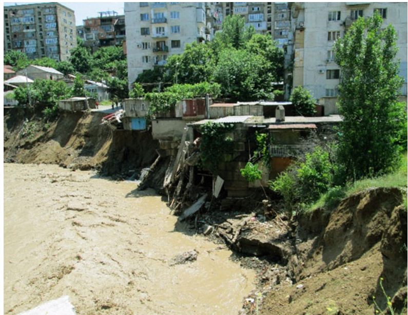
Fig. 7.12 River Bank erosion in Tbilisi city, 2015 (photo by G. Gaprindashvili)
