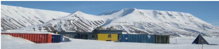
Fig. 4 UNIS Science Park in Longyearbyen. Site for assessing where CO 2 can be injected into a sealed subsurface formation consisting of porous sedimentary rocks. The black pyramid structure to the right shows the top of a well (Dh1)
