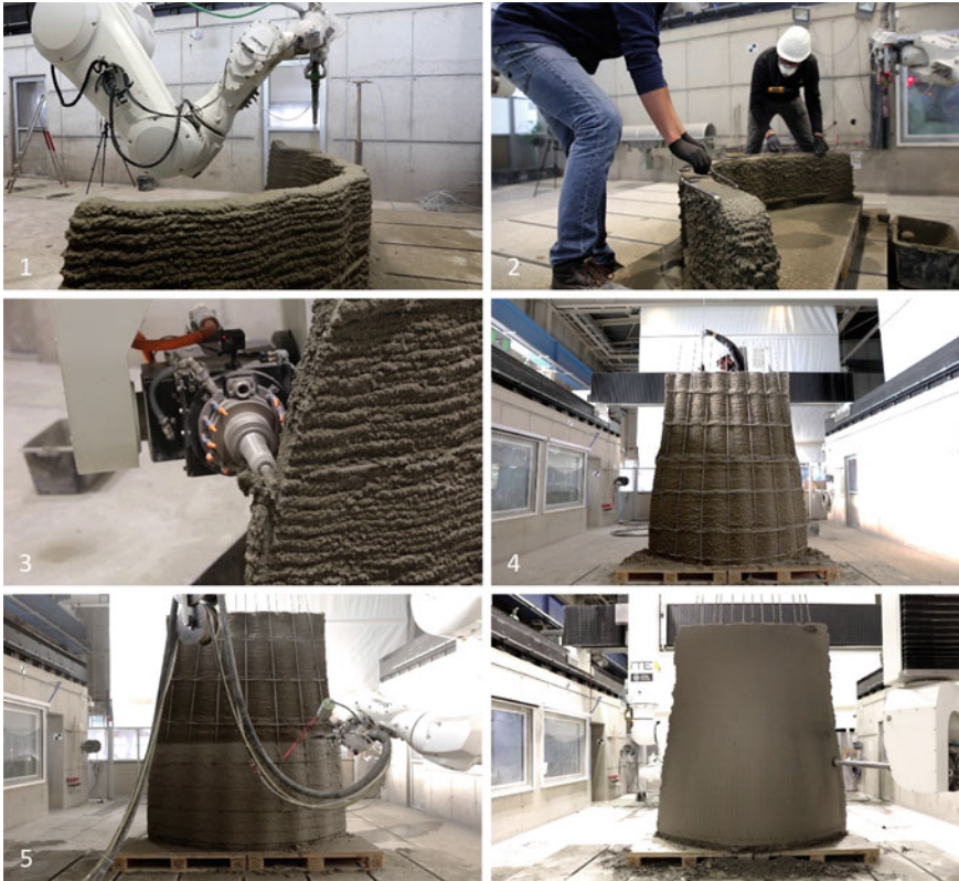
Fig. 2.12 Fabrication process; 1. Shotcrete 3D Printing of the wall; 2. manual placement of the pre-bent horizontal reinforcement; 3. precise cutting of the surface, while the concrete is still in the plastic state; 4. threading in the vertical reinforcement; 5. embedding the reinforcement by vertically spraying onto the printed structure; 6. final trowelling with a rotating plastic disc
