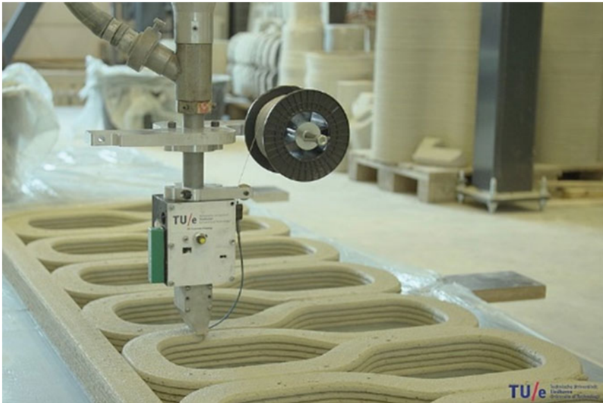
Fig. 2.3 Printing of a bicycle bridge element
