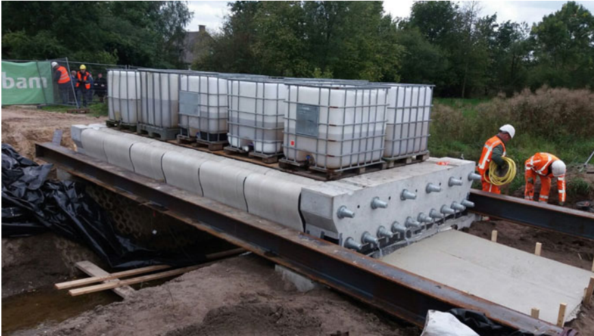
Fig. 2.5 In-situ testing of the bridge with water-filled containers
