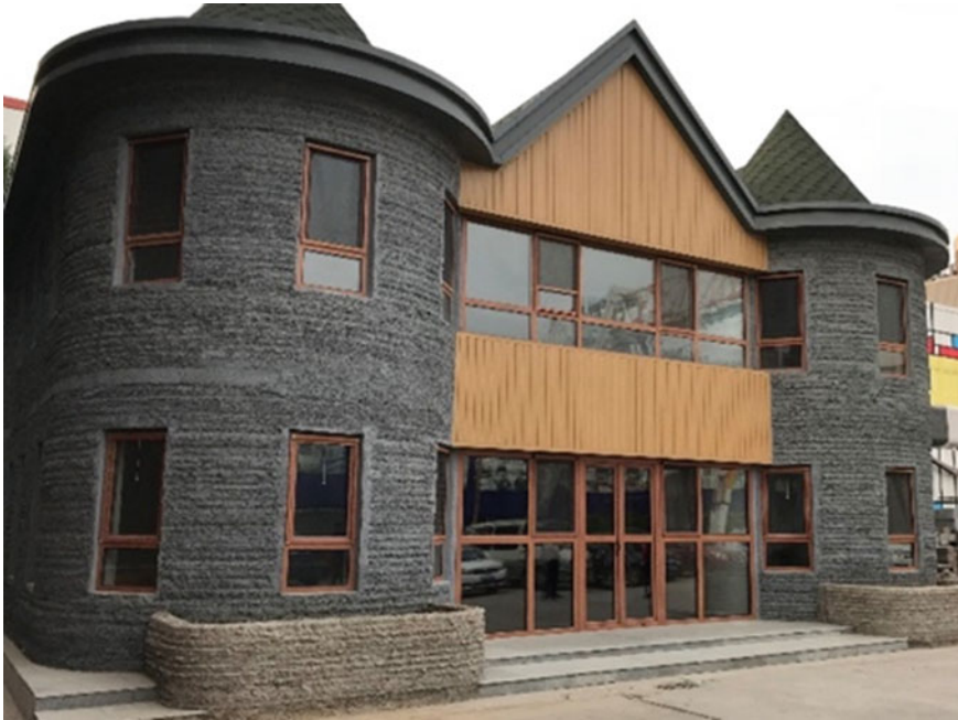
Fig. 2.22 The completed two-story villa
