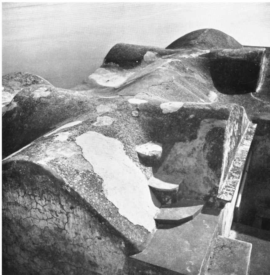
Fig. 5 The typical vaults that cover the traditional houses in the Sorrento-Amalfi peninsula in a photo by Roberto Pane (Roberto Pane Photo Archive, University of Naples Federico II)
