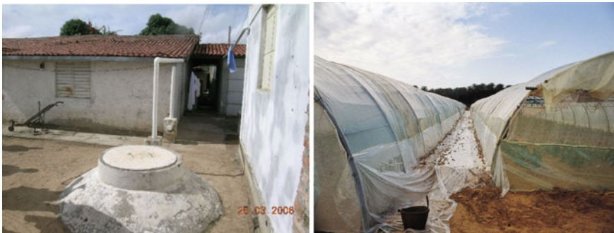
Fig. 4.1 Rooftop rainwater harvesting system (left) with underground storage in dry northeastern Brazil and greenhouse rainwater harvesting system (right) supporting protected vegetables in Alexandria area of Egypt (Credits: Theib Oweis, ICARDA)
