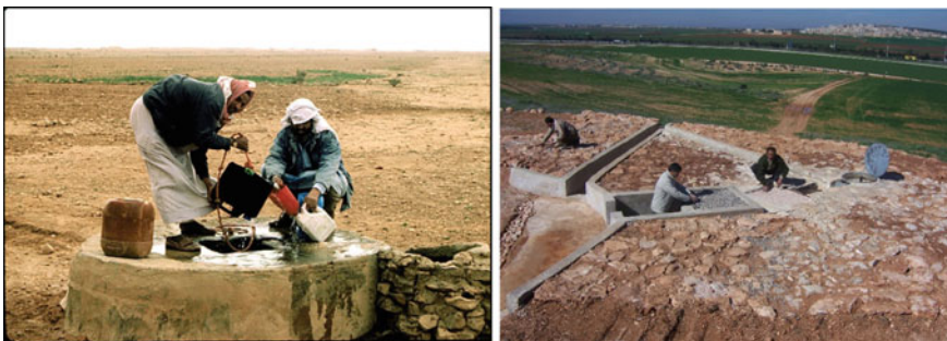
Fig. 4.2 Ancient cistern (left) still functioning and supporting communities in Matrouh, northern Egypt, and renovating an old cistern (right) with settling basin and filtration system at Tel Hadya, northern Syria (Credits: Theib Oweis, ICARDA)
