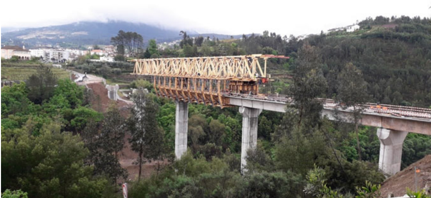
Fig. 2 Bridge over Tâmega River ( Source Infraestruturas de Portugal, 2020)
