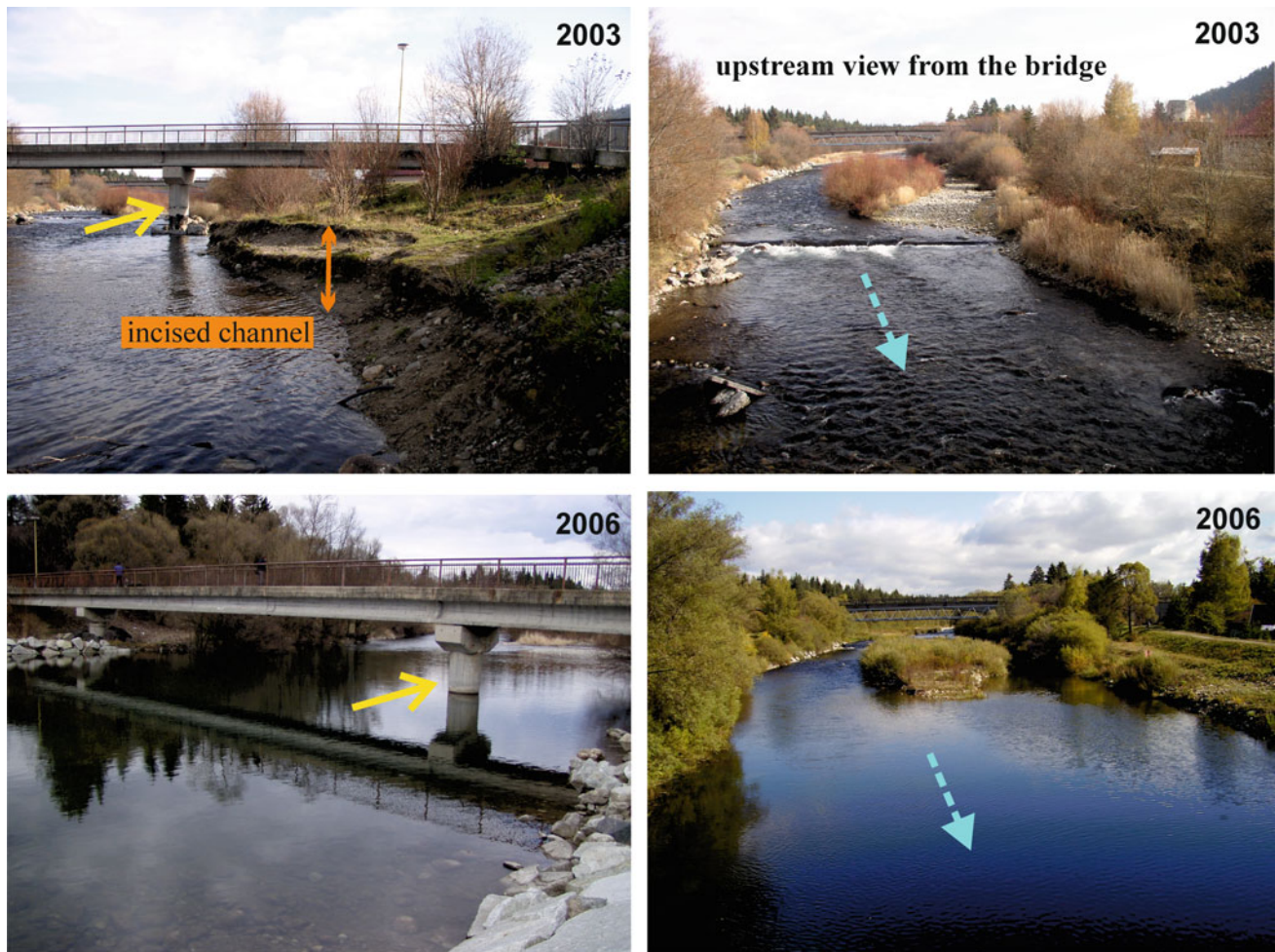
Fig. 15.5 The concrete grade control construction as a solution for the decreased groundwater level in 2003. The water marks on bridge pillar indicate the increased water level after channel regulation in 2006 during the third evolutionary phase. Photos A. Kidová, M. Lehotský
