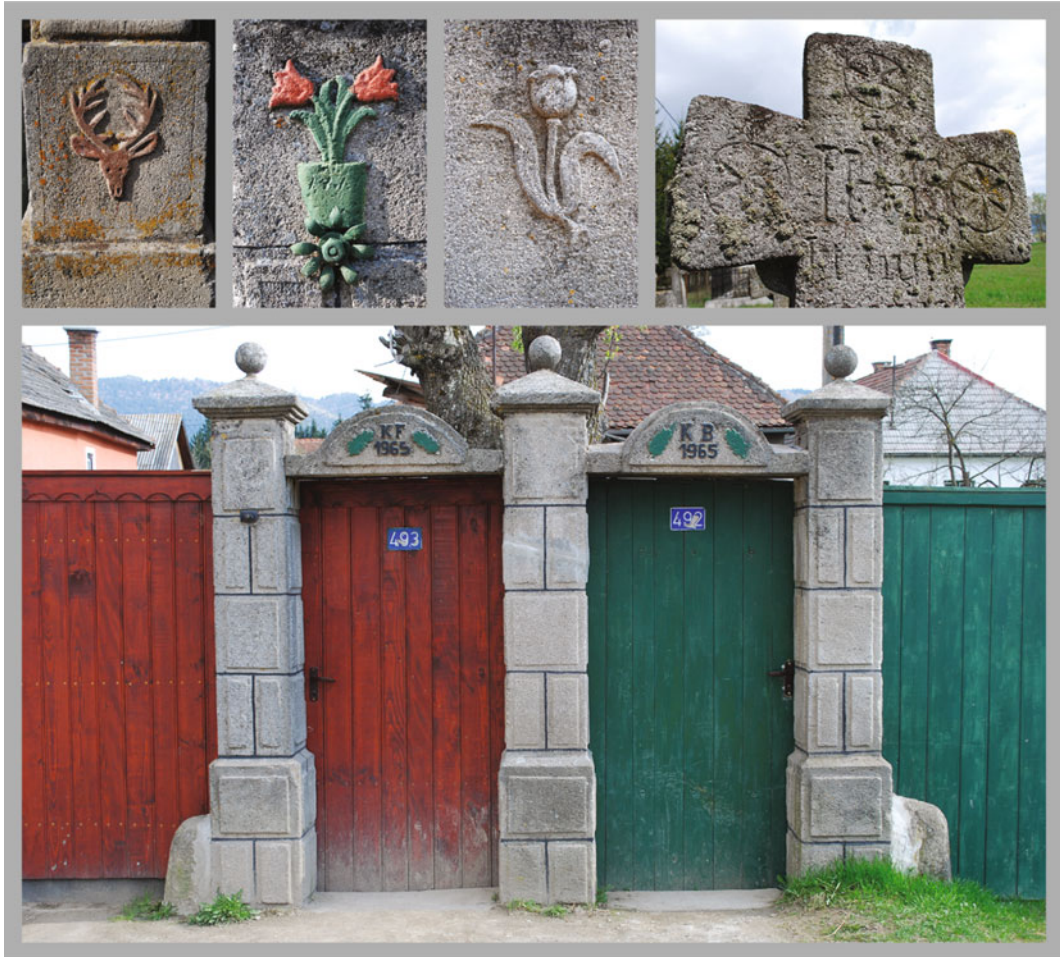
Fig. 17.5 In Lăzărești (Lázárfalva), Tușnad (Tusnád) and Tușnad Nou (Újtusnád, founded in 1822 after the great fire of Tușnad), the row of gates, gardens and houses carved into the relatively soft volcanic stone are spectacular and timeless. (The stone is dacite lava rock quarried
