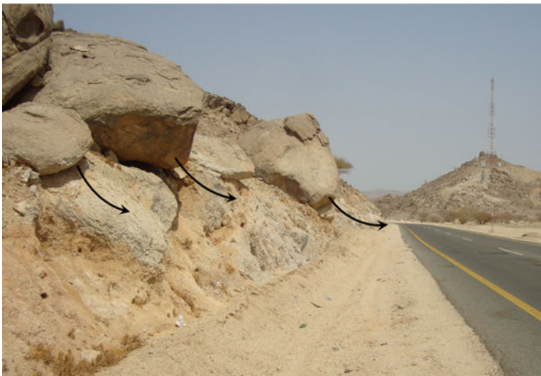
Fig. 7.1 Rocks susceptible to roll towards the road. (Al Saud, 2018)
