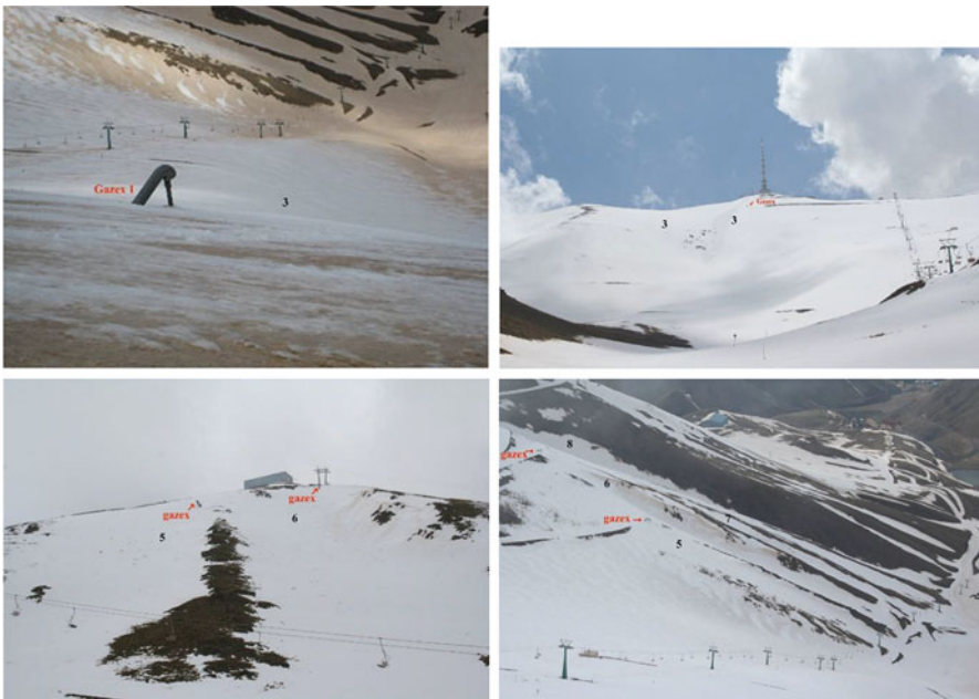
Fig. 23.14 Artificial avalanche release by using Gazex, Palandöken, Erzurum Province (Kurt, 2017)
