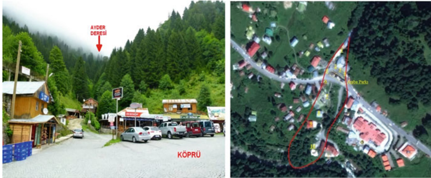
Fig. 23.27 Elements at risk according to (Çelik & Kurt, 2012)
