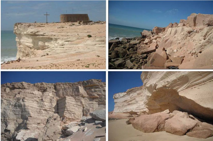
Fig. 9.5 Field photos shows Infrastructures destroyed by erosion (top right chapel and church – photo found on Google, other rubble photos and scree. (Source, Author, 2010)
