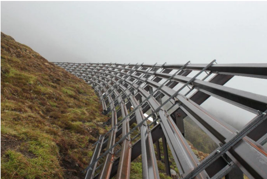
Fig. 23.12 Steel snow bridges in Trabzon (Photo: Anonym)
