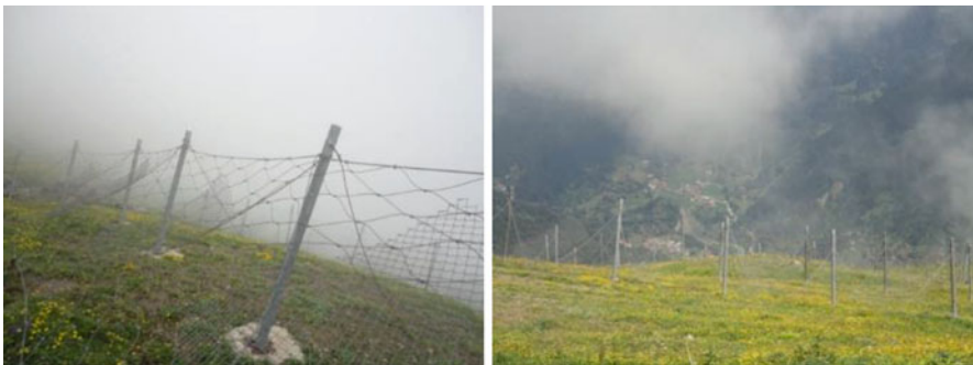
Fig. 23.10 Snow nets used as supporting structures in release zone, Uzungöl, province of Trabzon
