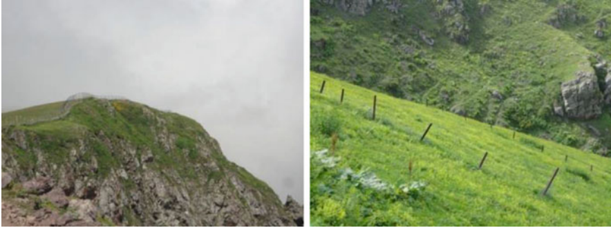
Fig. 23.11 Snow fences and mini-piles in Uzungöl, Trabzon
