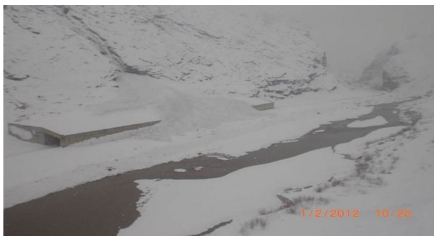
Fig. 23.16 Snow shed (206 meter long) in Province of Hakkari (Kurt, 2017)
