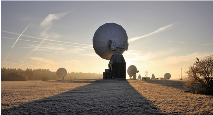
Fig. 11.4 IOT system in Ka-band with 13 m diameter antenna at Weilheim ground station
