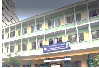
(b) Building of faculty
