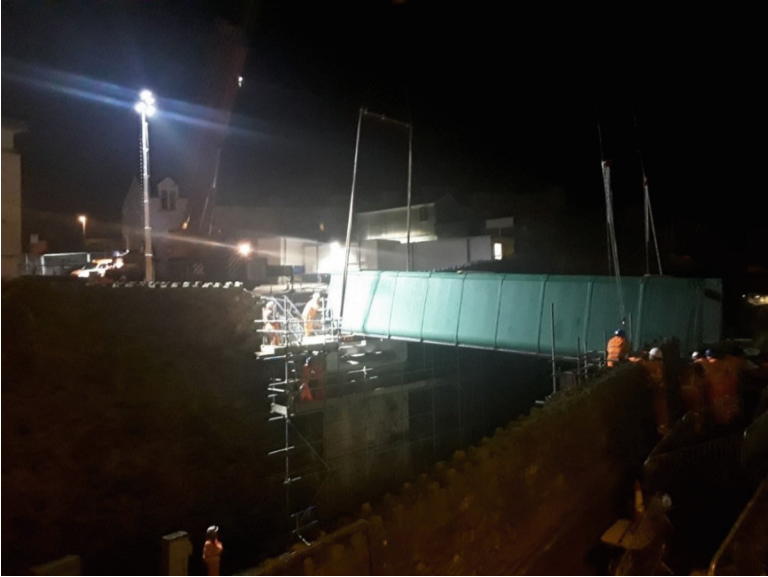
Fig. 8. Bridge installation and lifting operations
