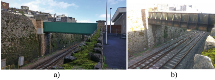
Fig. 1. Saxe Street footbridge, a) new replacement FRP footbridge, b) old wrought iron footbridge.
