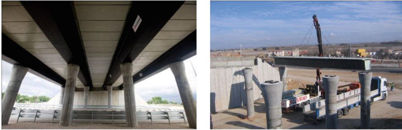
Fig. 1. Vehicular FRP bridges: M111 Madrid (Spain) freeway [13].
