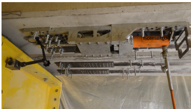
Fig. 6. Strengthening of the beams.
