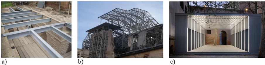
Fig. 1. Examples of FRP structures, a) temporary walkway, b) post-earthquake coverage, c) Glass-House.
