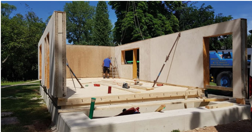
Fig. 3.4 House based on Miscanthus lightweight concrete, Luxembourg 2019
