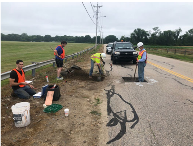
Fig. 8 Digging a hole for the irrigation box in the shoulder
