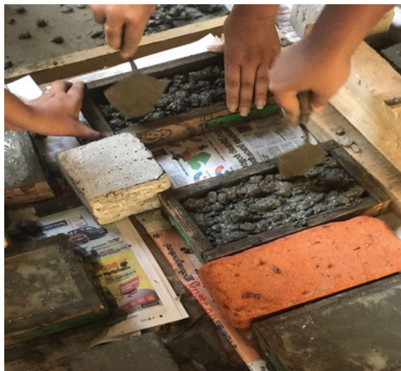
Fig. 1 Casting of paver block
