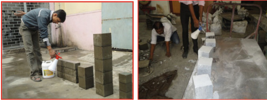
Fig. 1 Spraying of curing compound in progress
