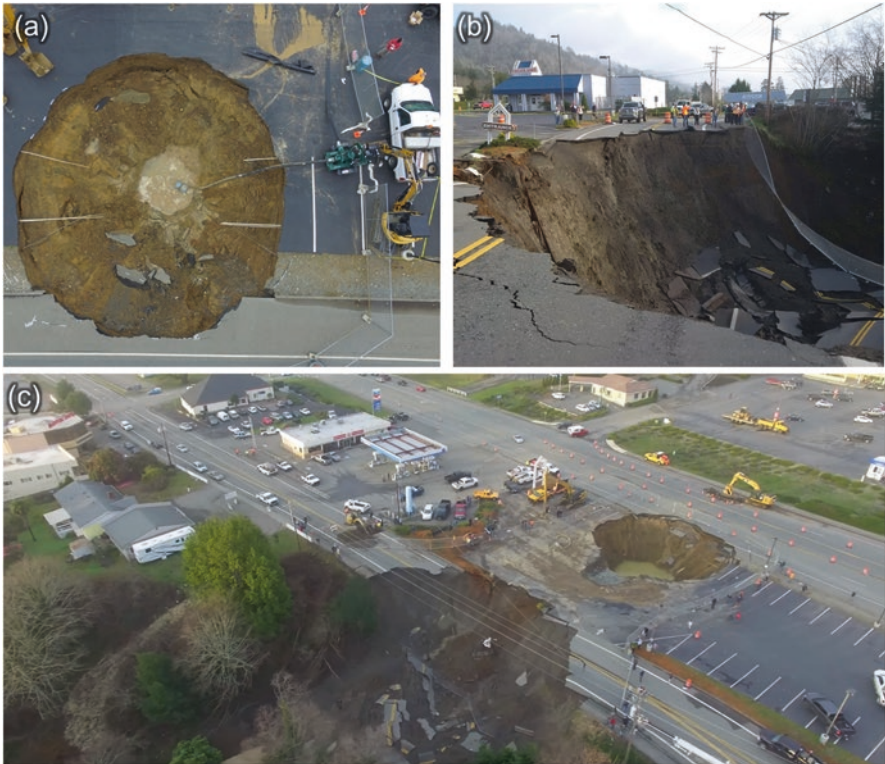
Fig. 5.13 A large sinkhole which formed in Harbor, Oregon, USA, in 2016, probably caused by preferential subsurface water flow down an infilled former valley (from upper right to lower left of image (c)) during heavy rainfall (Photo credits: (a, b), Oregon Department of Transportation, used under terms of Creative Commons Attribution 2.0 Generic license; (c) still from YouTube video by Kyle Rice, Triook Technology, Harbor, Oregon, USA (used with permission))
