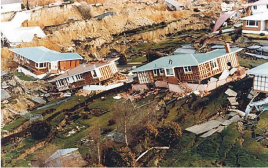
Fig. 5.7 Catastrophic slope failure in suburban Abbotsford, New Zealand, 1979. (Image from Hancox 2008; used with permission from Springer)
