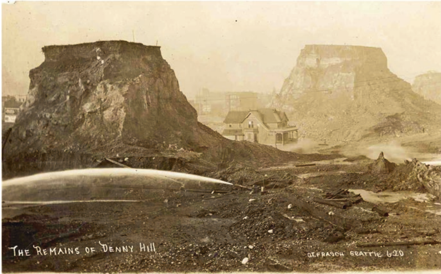
Fig. 2.9 Landscape truncation by complete removal of ‘Denny Hill’ in Seattle, USA (47.61 N, 122.33 W), in approximately 1910; public domain image by Shakespeare at https://commons.wikimedia.org/w/index.php?curid=16477653
