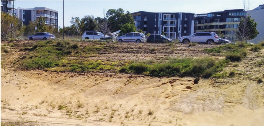
Fig. 5.4 Sheet and rill erosion of bare soil on a slope exposed by urban construction activities. (Photograph by Andrew W. Rate)
