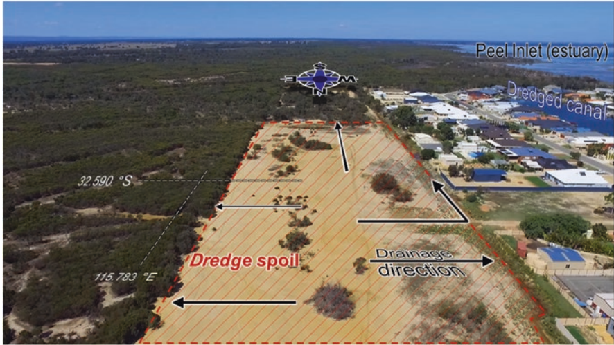
Fig. 2.7 South Yunderup, Western Australia ( -32.59 S, 115.782 E), showing a large area of dredge spoil in the foreground (with diagonal fill pattern) which has acidified due to the oxidation of pyrite and other sulphide minerals contained in the original estuarine sediment. (Photograph by Chris Yanicki (2017), used with permission)
