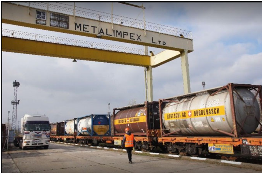
Fig. 31 Metalimpex terminal in Stara Zagora
